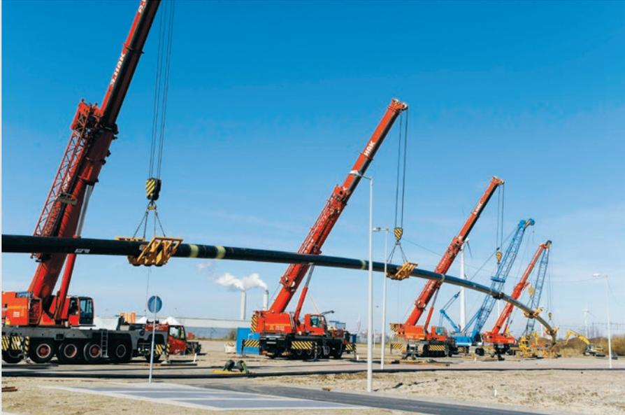
*FW STEEL-CASED PIPE-IN-PIPE 500/70/700 for a construction project in the Netherlands.
