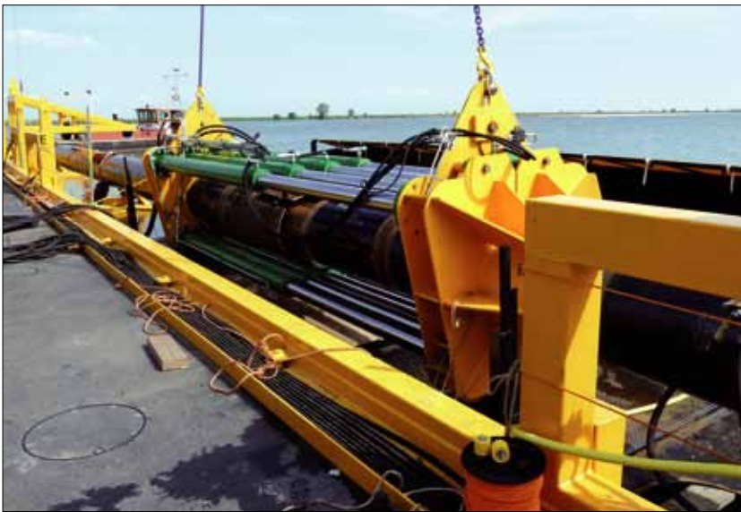
Figure 4. Pipe-laying pontoon with hydraulic pre-stressing device
