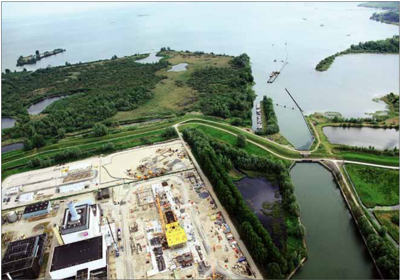
Figure 2. Dyke-crossing with horizontal directional drilling (HDD)
