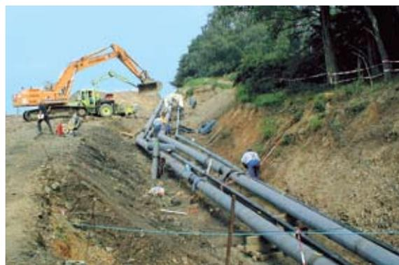
*FW SAFETY PIPING DN 100/125, DN 300/350, 3,600 metres, transporting kerosene and diesel oil*
